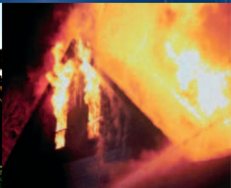
Fire in a residential building caused by a direct lightning strike
